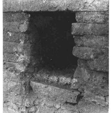
Fig. 192 b . S. Pietro in Vincoli, North clerestorey, beam hole for aisle roof, church A
